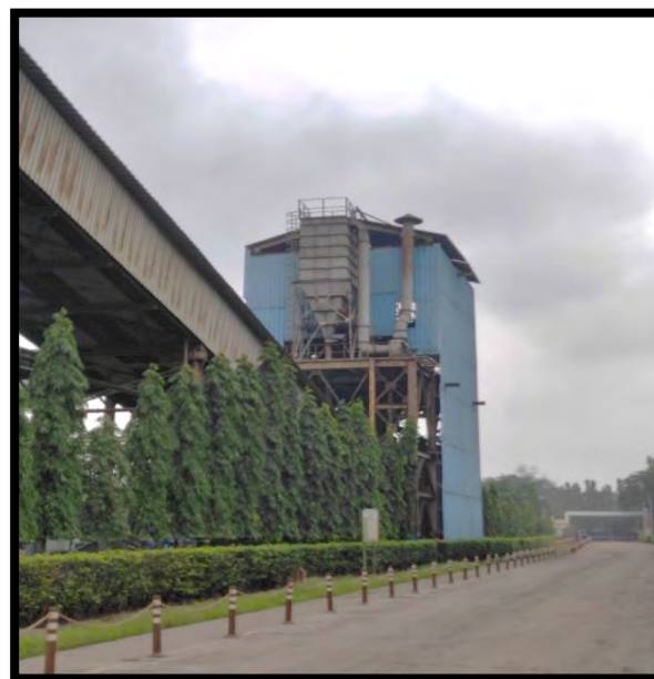
Dedusting Units in Coal Handling Plant
