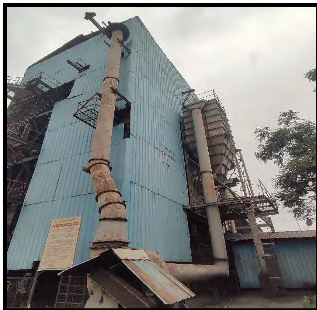
Dedusting Units in Coal Handling Plant
