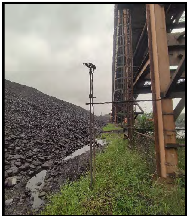
Water Sprinklers in Coal Stock Area
