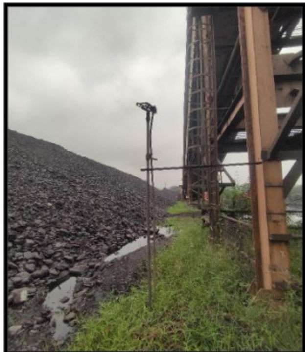
Water Sprinklers in Coal Stock Area
