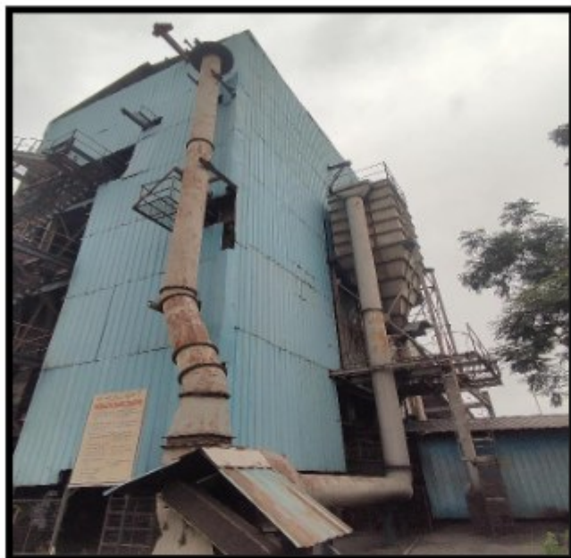
Dedusting Units in Coal Handling Plant
