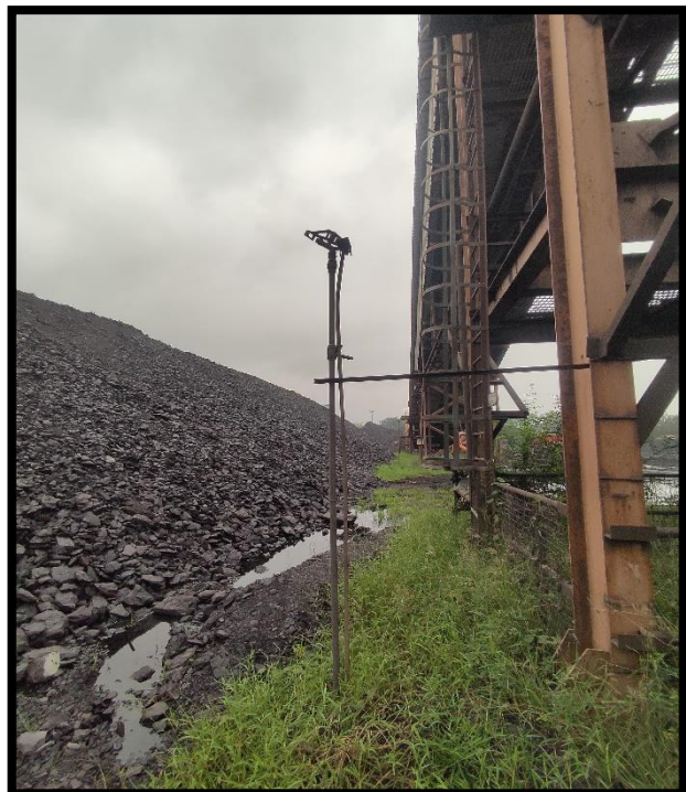
Water Sprinklers in Coal Stock Area
