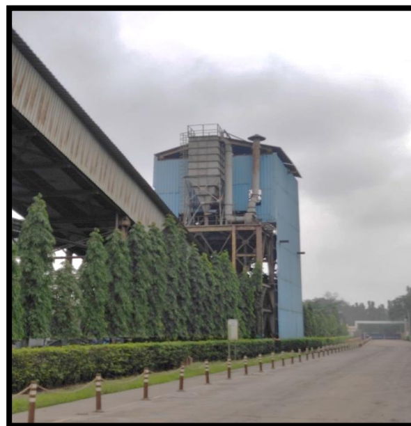
Dedusting Units in Coal Handling Plant
