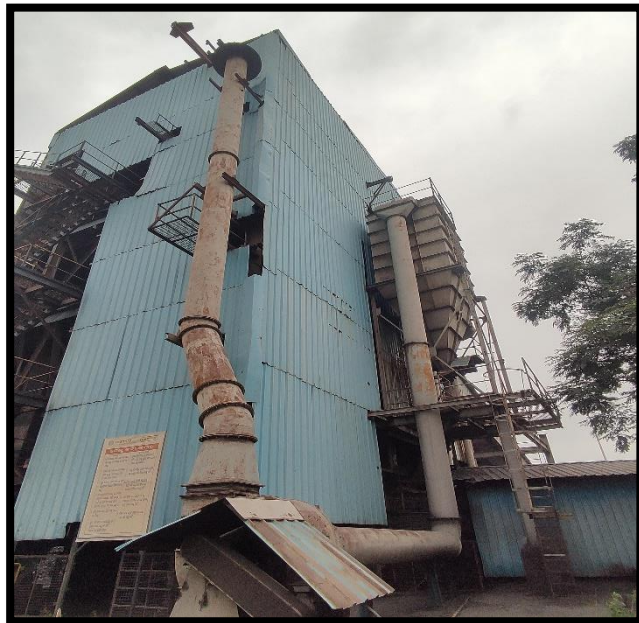
Dedusting Units in Coal Handling Plant
