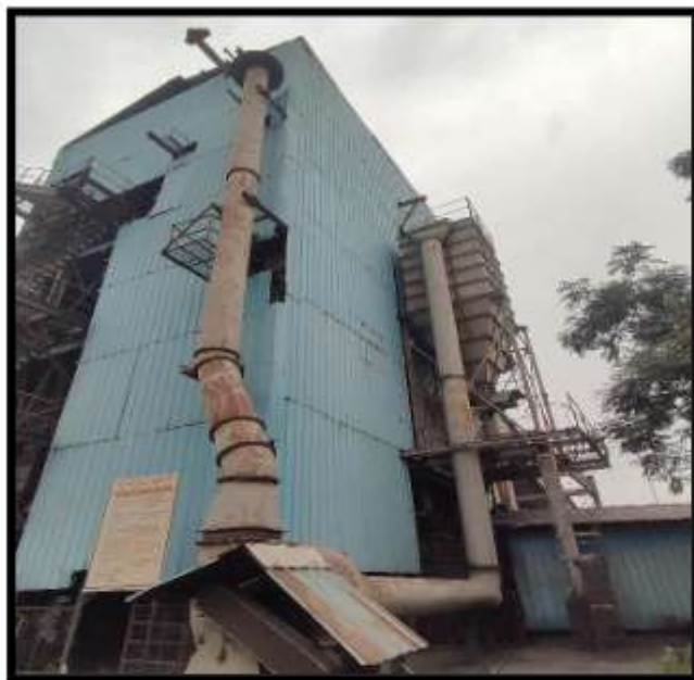
Dedusting Units in Coal Handling Plant
