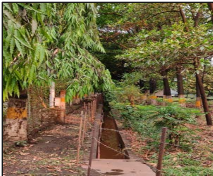
Drainage System to Collection Surface Runoff
