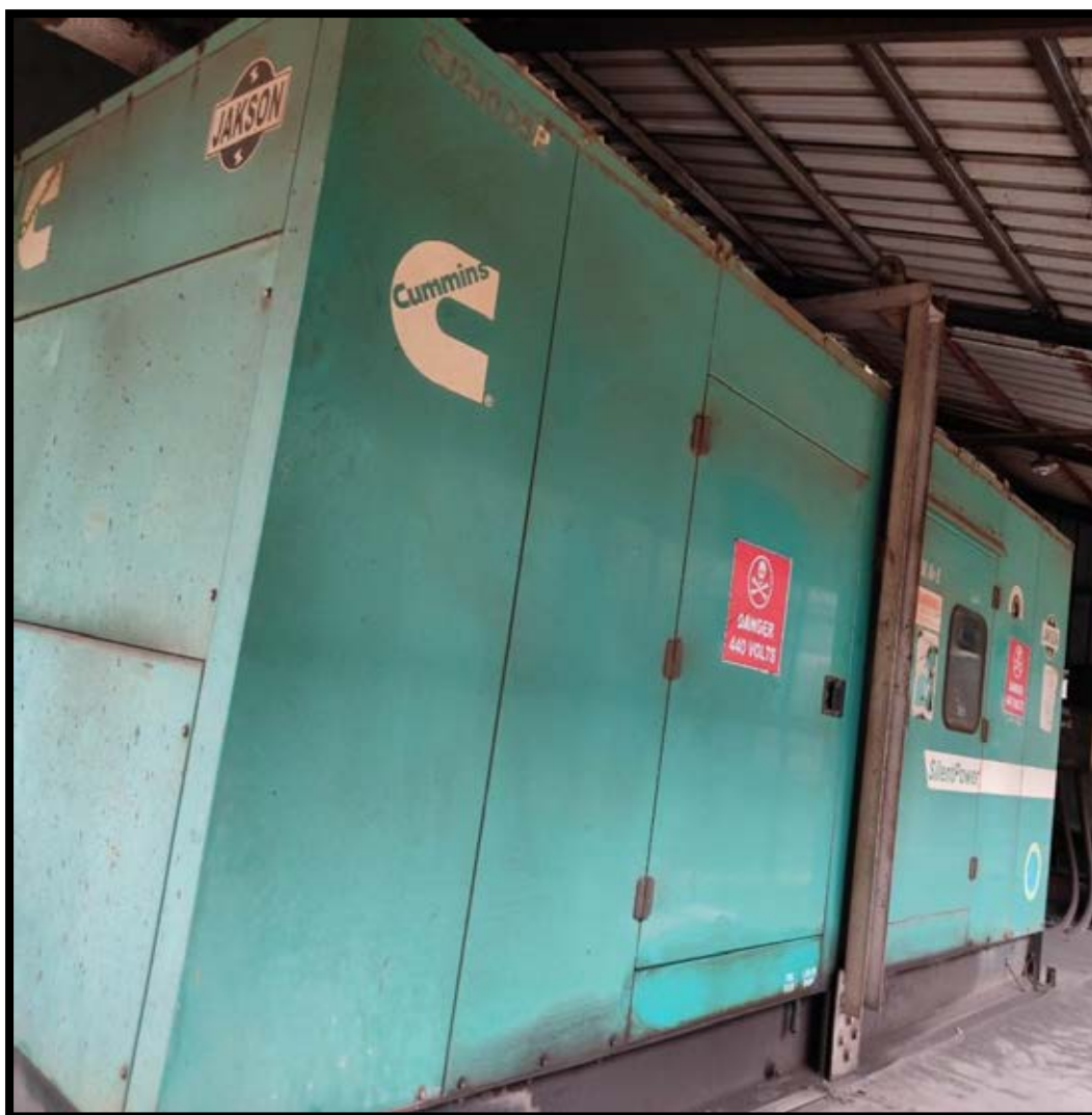
DG Set with Acoustic Enclosure
