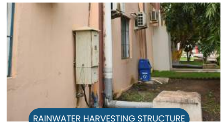
RAINWATER HARVESTING STRUCTURE
