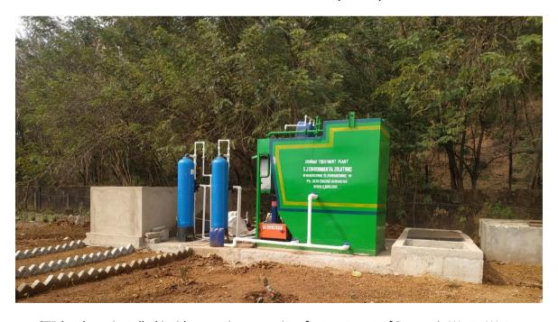
STP has been installed inside our mines premises for treatment of Domestic Waste Water
