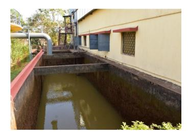
ETP OF 600M3/HR CAPACITY INSTALLED INSIDE MINES FOR TREATMENT OF HEXVALENT CHROMIUM (CR6+) WATER .
